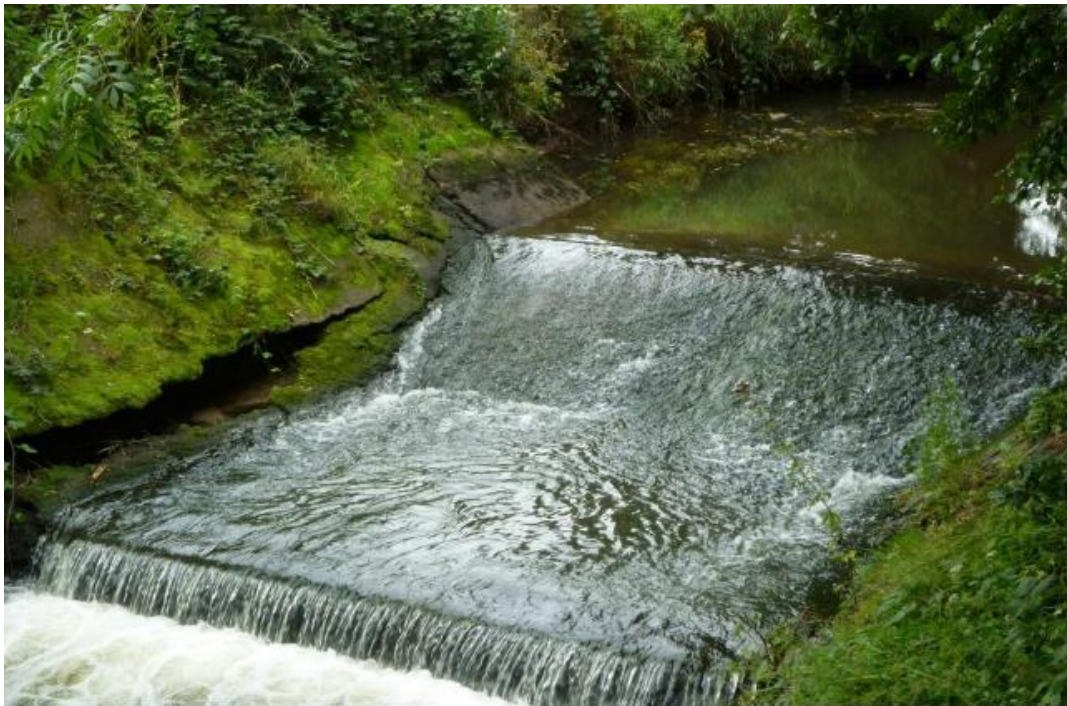
Photo 1 - Harpers Weir on the River Teise (Medway catchment, Kent), which was recently removed revealing thirteen new gravel riffles, additional spawning habitat for the native brown trout.
