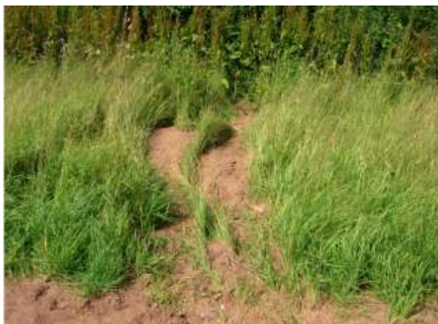
Photo 6 Breaching of buffer strip
