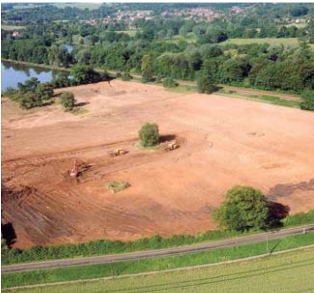
Marsh Farm construction
