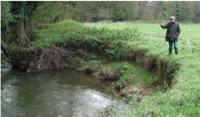
Eroded river bank – disease and poor management of bankside trees can exacerbate bank failure, erosion and increase the amount of fine sediment that enters the river.
