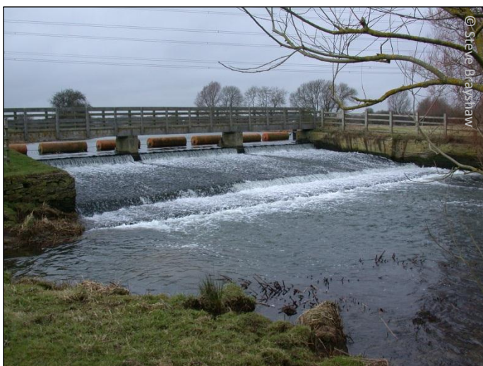
Fig 19. Water Newton Weir is currently a barrier to fish and eel passage
