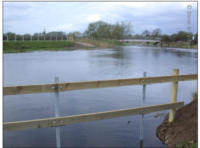
Fig 12. Cattle drinker front fencing showing angle iron uprights used to penetrate the hard river bed.
