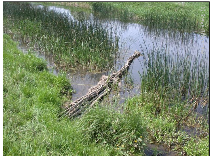
Figs 3 & 4. Faggot deflectors used to pinch the channel and to consolidate existing and encourage future siltation
