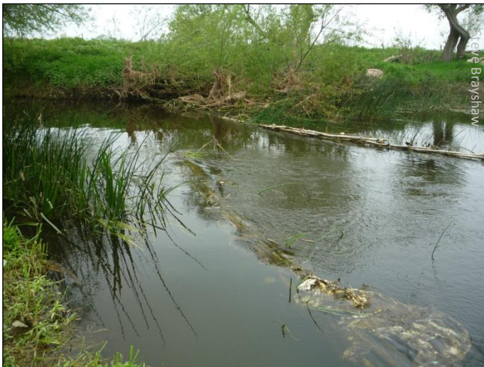
Figs 3 & 4. Faggot deflectors used to pinch the channel and to consolidate existing and encourage future siltation
