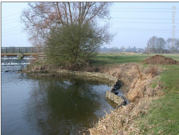
Fig 9. Ash spiling used to protect bank toe
