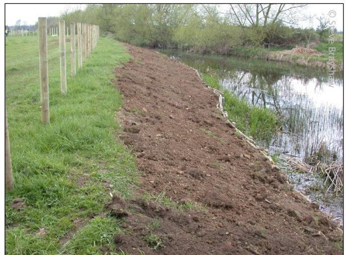
Fig 10. Eroded bank reprofiled behind spiling
