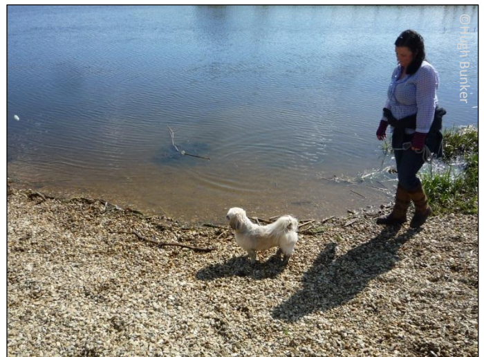
Fig 14. After: the repaired "dog-dip"
