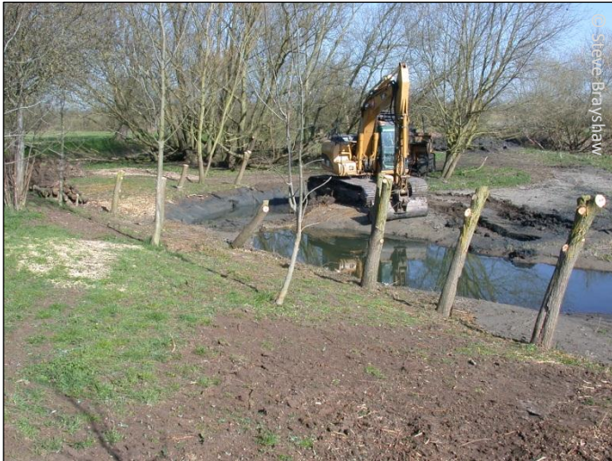
Fig 7. Lower refuge pool under construction
