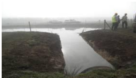
The new connection between the reedbed and the Thames
