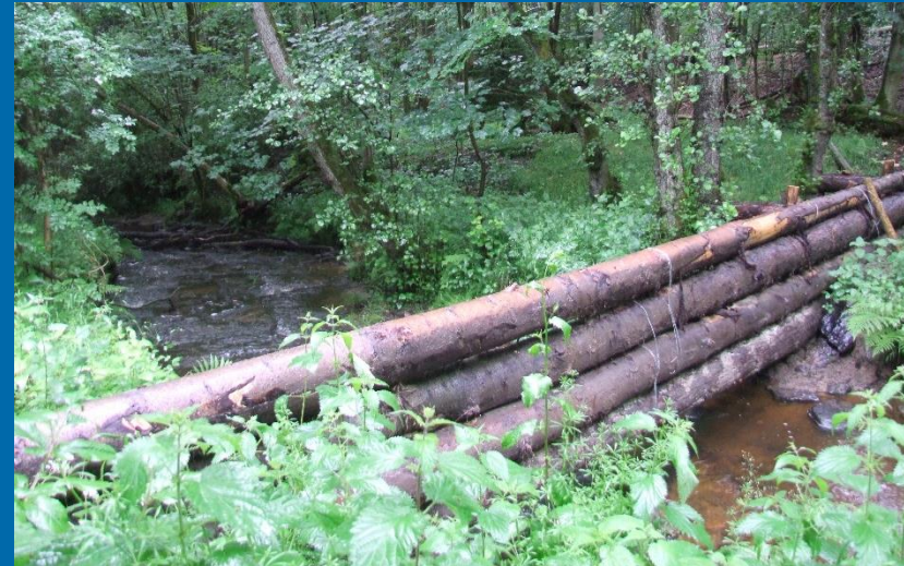
High level timber dams
