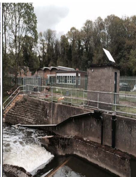
The completed eel ramp
