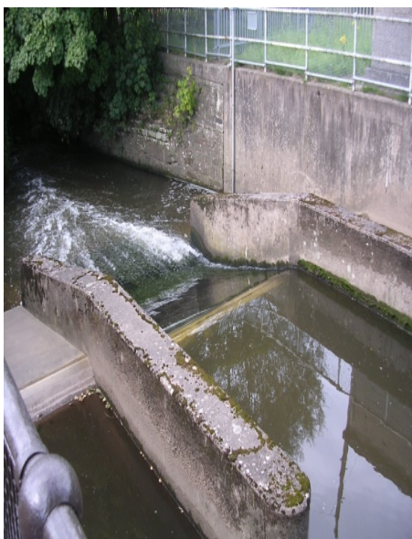
The existing gauging weir at Wilmslow
